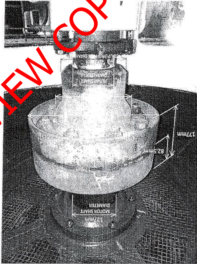
Existing coupling dimensions between pump and motor (vertical installation)
