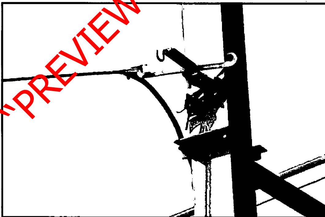
Termination bracket with split tube protection of OFC
