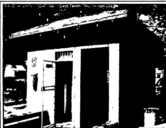
Asset: 02AF098K - View from : Unspecified Date: 04-Apr-2013 File No: 55010236 (1/6)
