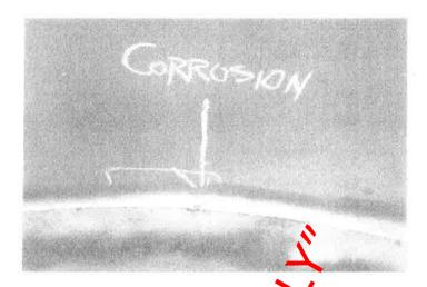
1.1.3 The water drain pipe bracket is keited directly on the sump. Replace water drain pipe bracket welded directly on the floor with bracket welded on pads.
