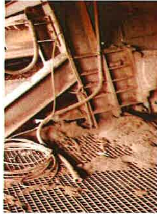
Figure 4: Inner chute treatment point not connected for dosing plant on CV 114.
