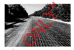
After the form sections have been properly aligned over a certain distance, they are secured by means of stakes. As the side forms serve as the reference for guiding the vibratory screed, the tolerances for the evenness shall not be exceeded. To accurately place he forms, a rigid template having the same width as the concrete pavement must be available on site, so that it can be checked at any time whether or not the form sections are set up parallel.
