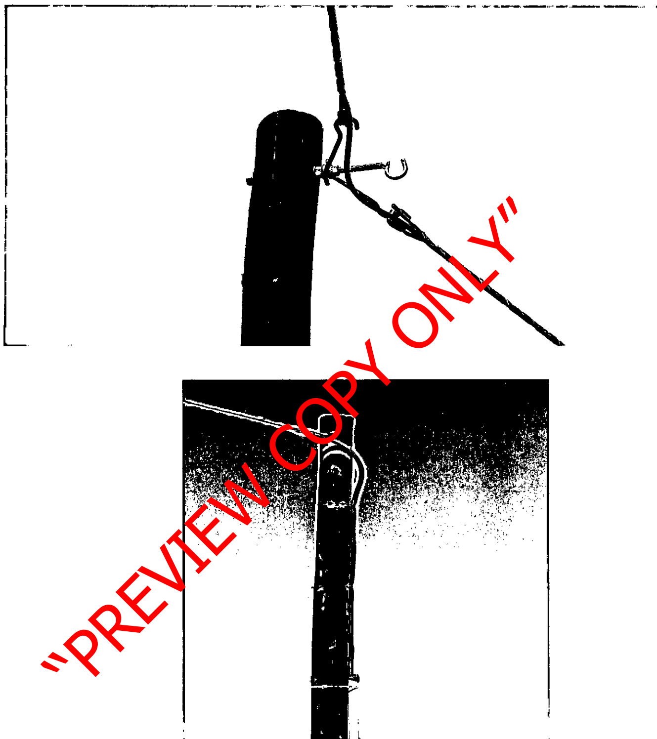
Correct method of OFC termination on pole Clause 5.9.4)
