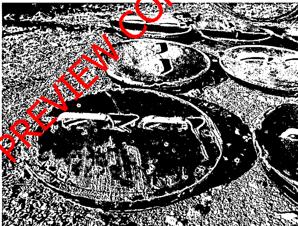
Concrete filled manhole covers for GRP manhole (clause 6.1.4)
