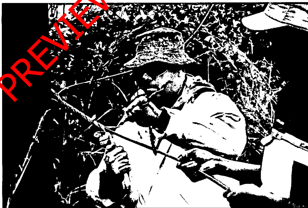
Cable termination by means of dead-end (Clause 3.7)
